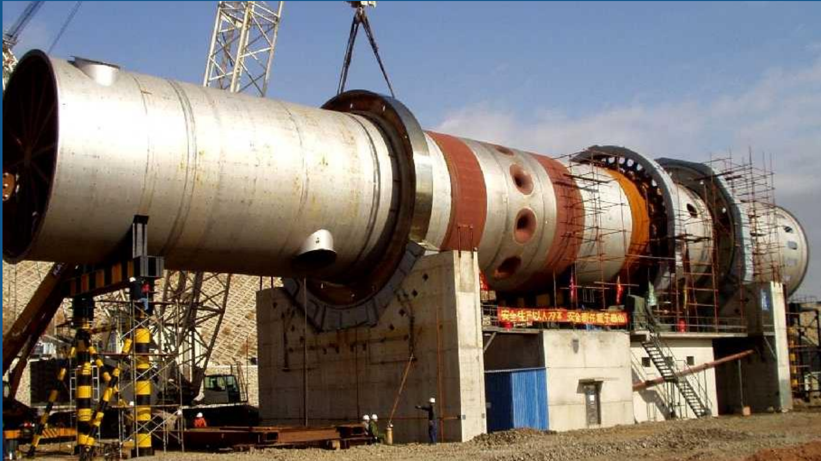
ATP Processor in Construction - Outer Shell Erected. Commissioning Fall 2009.
