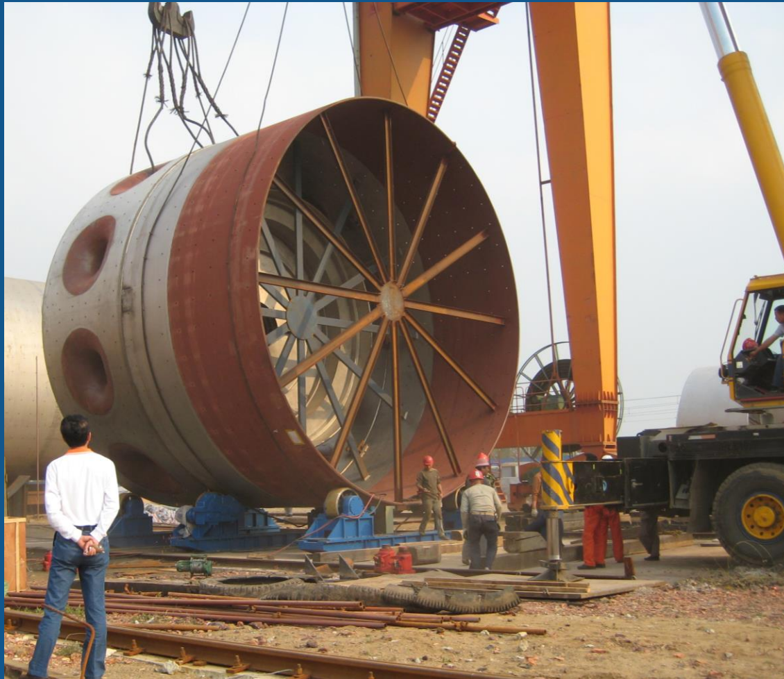
ATP Processor Erection in China September 2008
