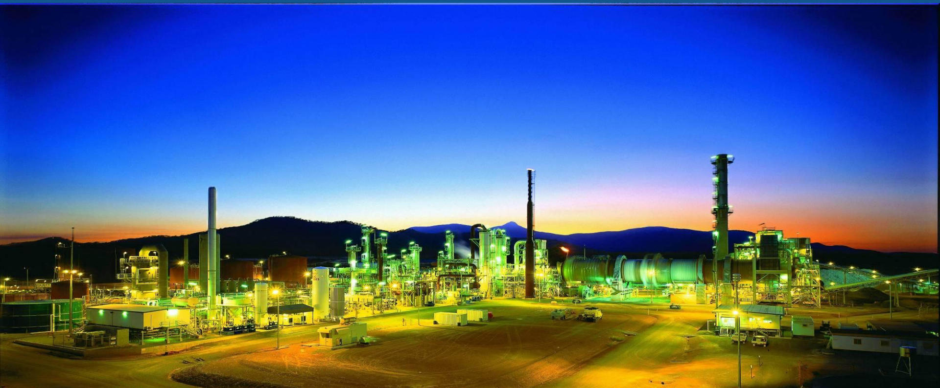
ATP Plant and Upgrader
